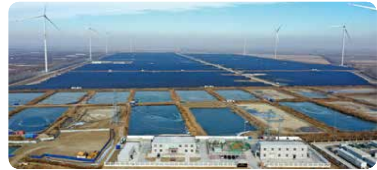
Ninghe wind power project in Tianjin
