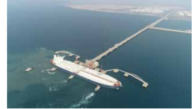
After resumption of work and production of SDIC Oil & Gas Terminal Yangpu, the first 300,000-ton oil tanker was performing loading and discharge tasks
